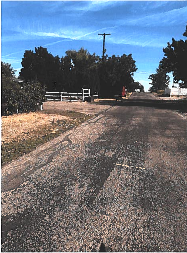
Neighborhood view in front of 924 N. 52nd Street
